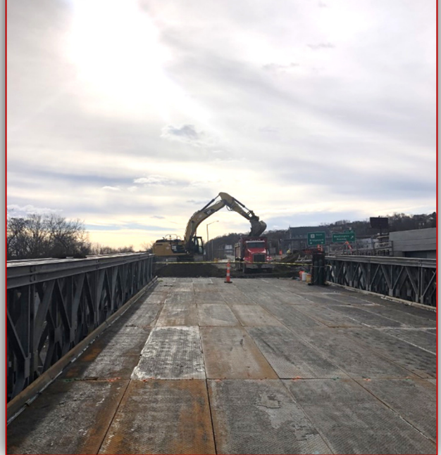
Removal of Temporary Bridge 1, Abutment 1
